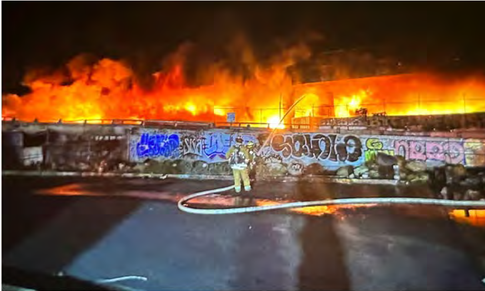
A fire along Interstate 10 near downtown Los Angeles, Nov. 11, 2023.
